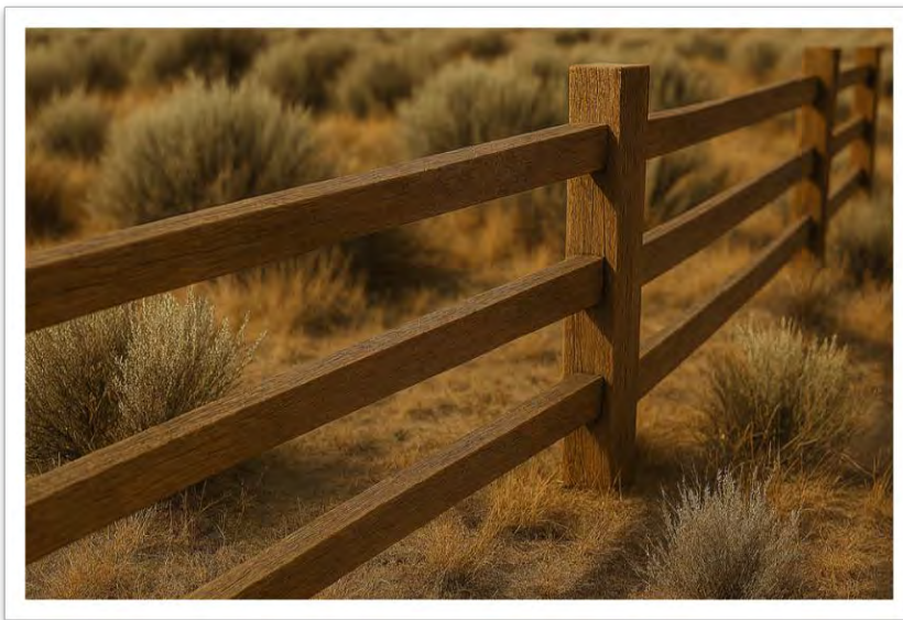
Figure 6: Split-Rail Fence Example
